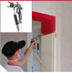
AirCoat guns for high-yield painting work on the construction site. Light, and incorporating perfect ergonomics (with ACF 3000
